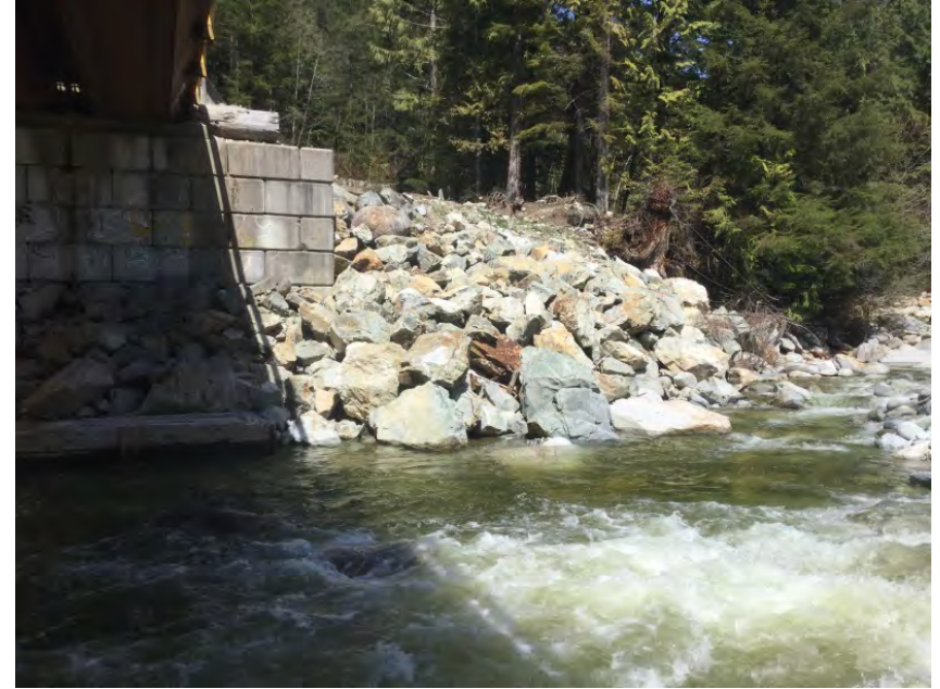
Upstream right bank riprap
