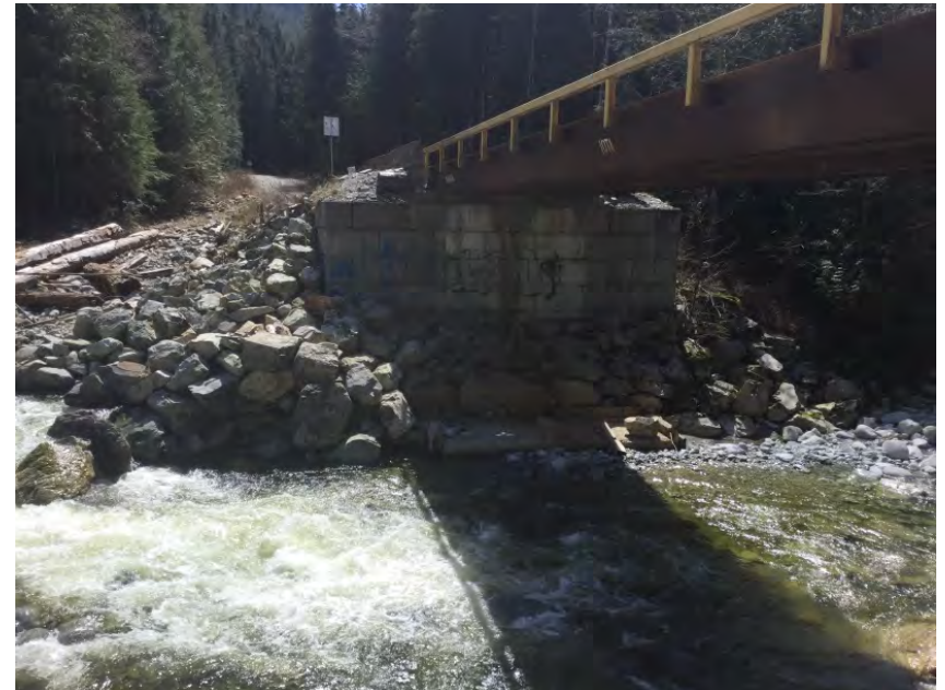
Left Bank Abutment when facing downstream
