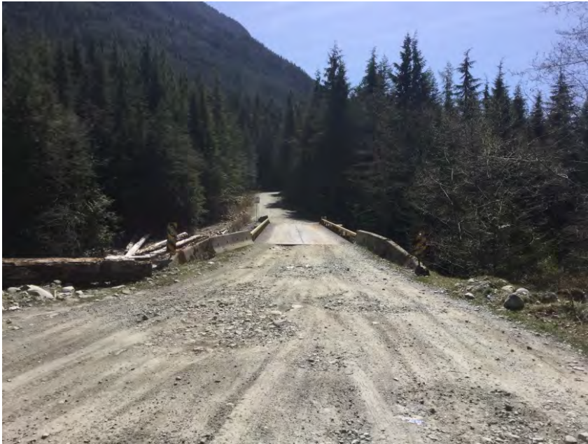
Approach from Right Bank when facing downstream
