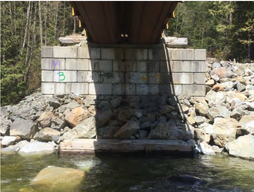
Right Bank Abutment when facing downstream
